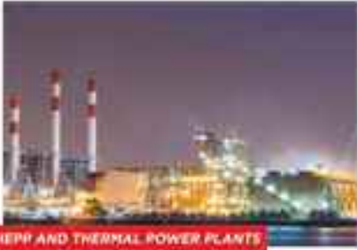
HEPP AND THERMAL POWER PLANTS
